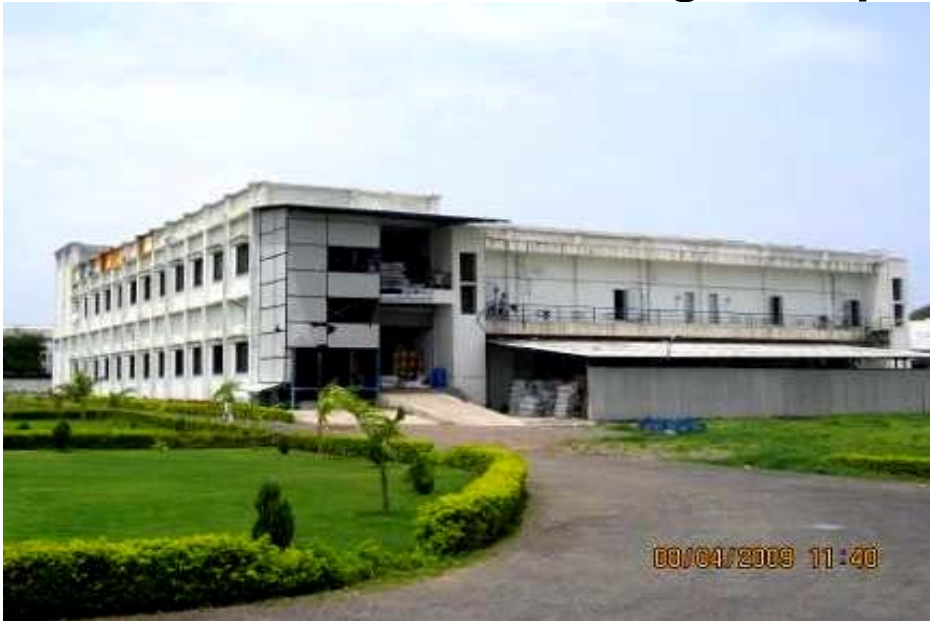
Factory surrounded by extensive grounds
